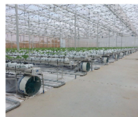
Green House Slab
